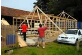
Vince Smith at work on frame and roof trusses
