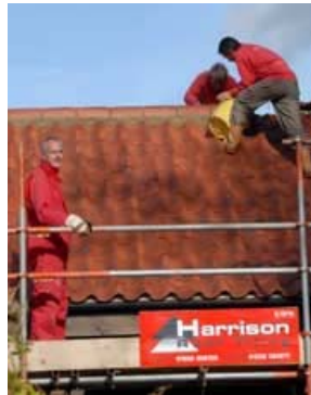
Tim Harrison supervises the fitting of the ridge tiles
