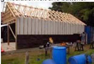
Fitting the cladding
