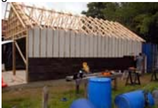
Fitting the cladding
