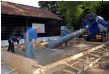
Ley Plant at work on the base
